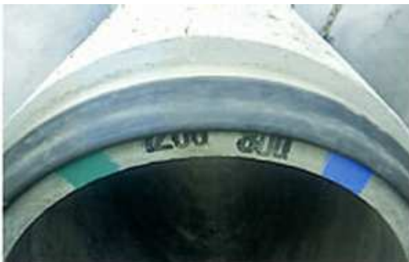
View of correctly positioned seal
