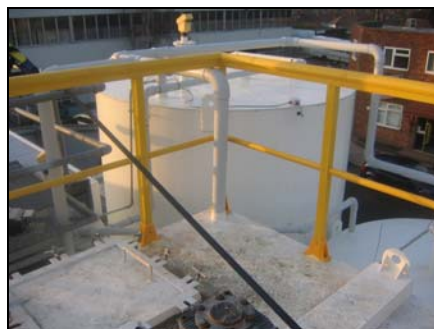
Yellow handrail system
