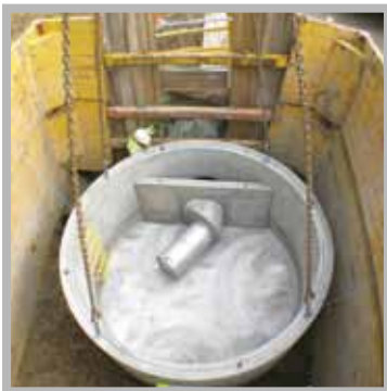
3000mm wide wall chamber complete with a separate bolted headwall and CX Hydro-Brake®
