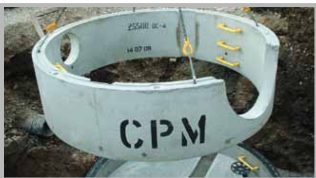
2550mm sectional installation, upper ring with half formed hole for 900mm pipe and formed inlet hole
