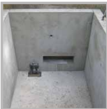
Once-piece chamber with inlet and outlet holes
