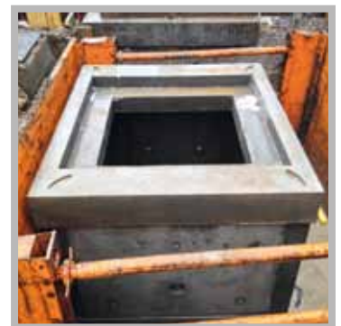
Flat pack chamber complete with rebated cover slab for access cover
