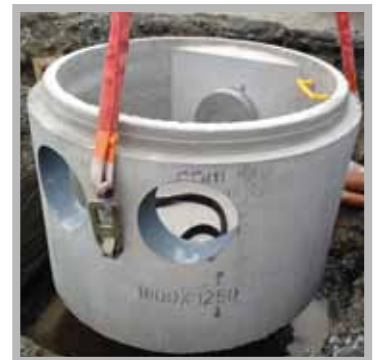
1800mm sealed chamber complete with Optimum Hydro-Brake®
