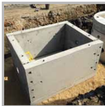
Flat pack installation
