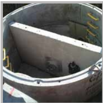
2550mm wide wall chamber installed complete with Hydro-Brake® and penstock on weir wall.
