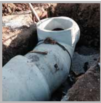
900mm off 900mm mid entry manhole
