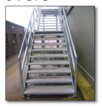
Anti-Slip Tread Covers are a simple and cost effective way to provide superior slip resistance on stair ways. They are extremely durable and completely corrosion resistant. They have a contrasting nosing for high visibility. Tread covers can be cut and drilled if required to your exact specification. Internal and external adhesives are available to complete the installation. Landing areas also available utilising our fibreglass plate.
