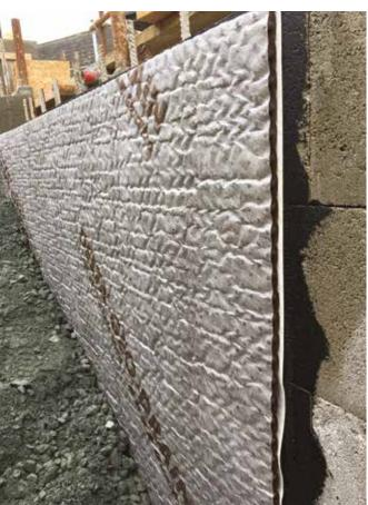
"Tanking", provides protection against ground water ingress by applying a waterproof material to the internal or external walls and floor slab of a basement or underground structure forming a barrier between the structure and any groundwater present.
