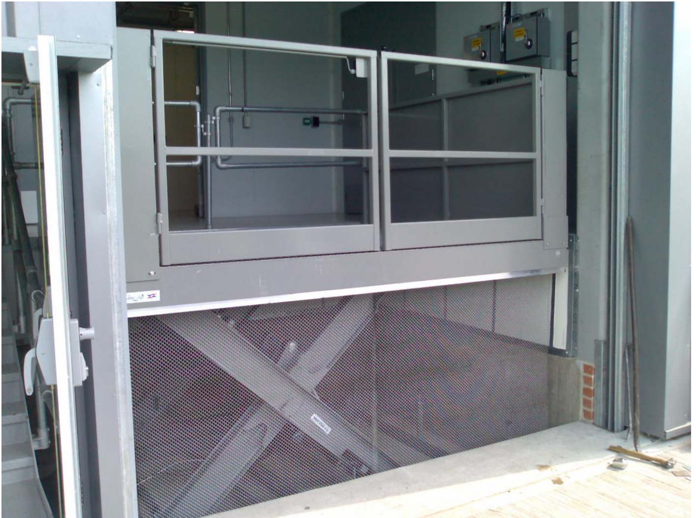
Split Level Goods Elevator Platform Lift
