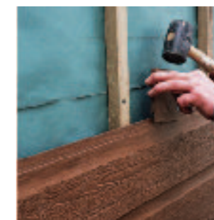
Use an off-cut and hammer to fully connect the planks
