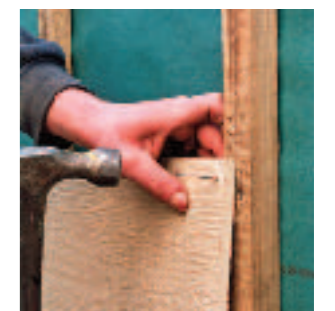
Plank cuts painted – use stainless steel ringshank nails
