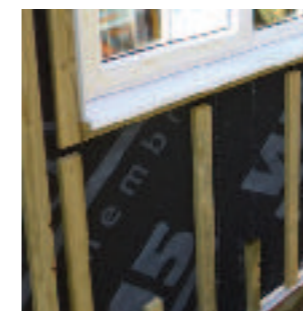
Battens with airflow around windows
