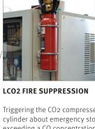
Triggering the CO2 compressed gas cylinder about emergency stop, exceeding a CO concentration value or one temperature increase in the test room.
