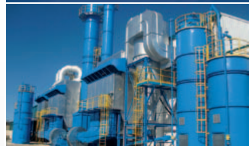
Travelling medium pressure – off line – cleaning
