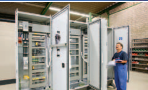
Control panel construction
