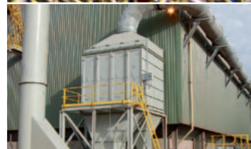
Compressed air – on line – cleaning
