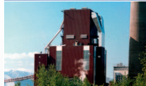
Compartmentalised compressed air – off line – cleaning
