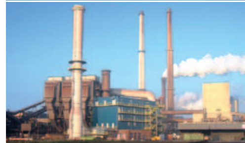
Travelling compressed air – off line – cleaning
