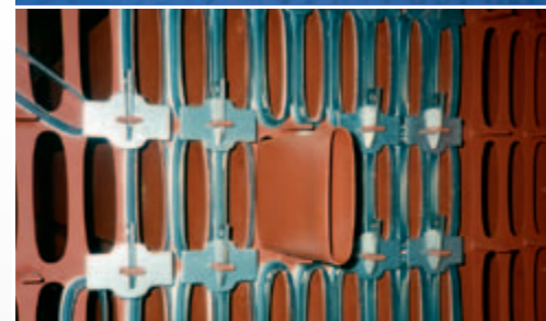
Perforated plate with flat-tube cooling elements
