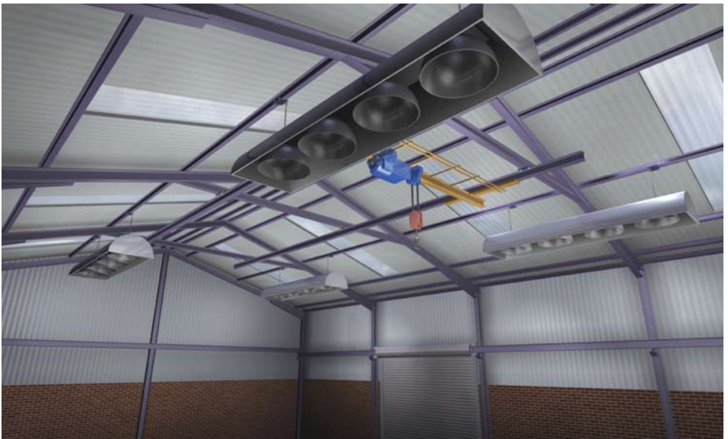
Hanging of industrial lighting systems
