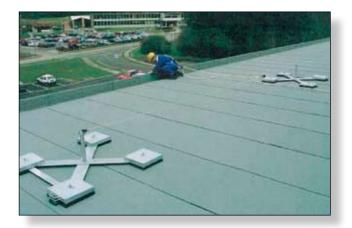
To be classified as restraint, the position of the **WIREANKA** and the length of the lanyard must ensure it is not possible to approach within 500mm of a roof edge or other opening.
