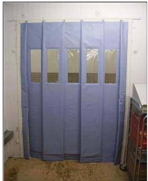
From inside the cold room
