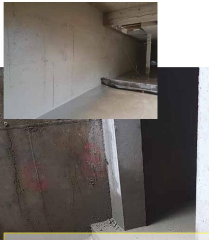
A Type C Cavity Drain system is made up of cuspated membranes which are applied to the walls and floor of a basement with a channel incorporated at the wall/floor junction. The cavity drain membrane allows any water ingress to filter down to the slab and find its way to the perimeter channel. The channel directs any water ingress to a sump pump or agreed drainage points which is situated below the slab (floor). The sump pump chamber will then remove any water ingress to the ground level drains.
