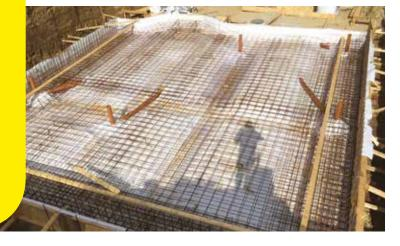
DualProof is a Type A waterproofing pre-applied, sealed two layer highly flexible PVC membrane laminated with a non-woven PP-fleece, composite waterproofing membrane which forms a permanent mechanical bond with freshly poured concrete preventing the tracking of water between the waterproofing membrane and the concrete sub-structure.
