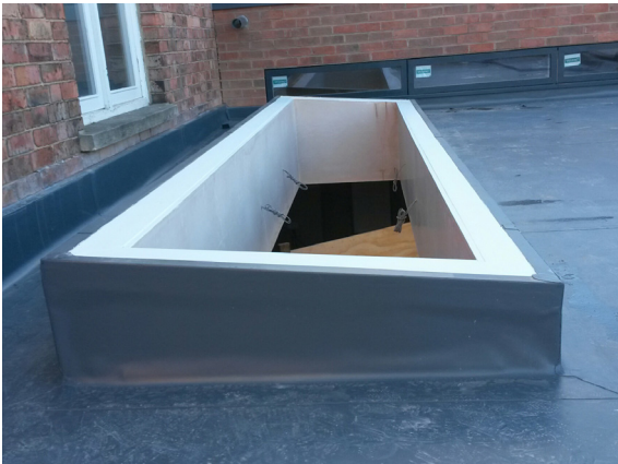
Upstand complete with weathering.
