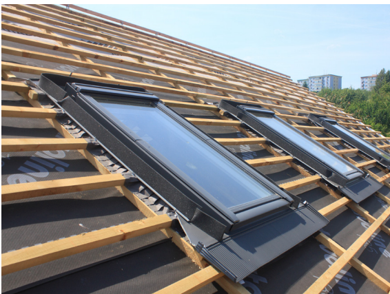
Roof window install prior to flashing and tiling.
