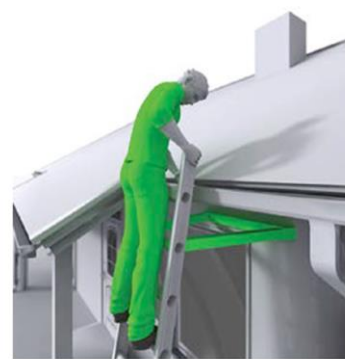
Figure 4 Correct – use of a stand-off device to ensure a strong resting point. Do not rest a ladder against weak upper surfaces such as glazing or plastic gutters. Follow the manufacturer's instructions
