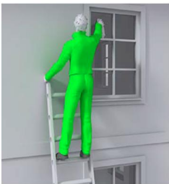
Figure 2 Correct – user maintaining three points of contact (means of securing omitted for clarity)
