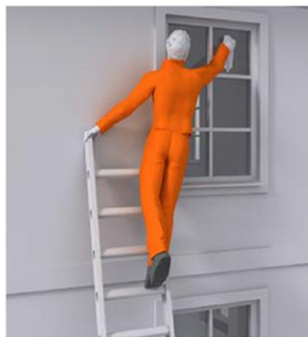
Figure 3 Incorrect – overreaching and not maintaining three points of contact (means of securing omitted for clarity)
