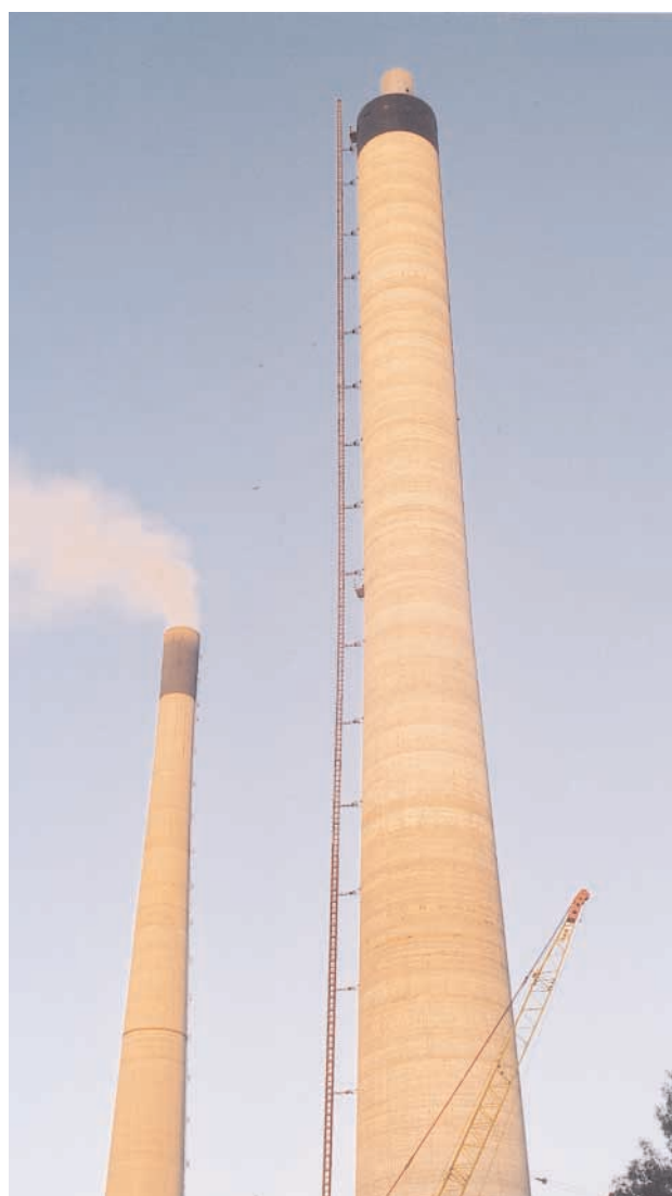
The Alimak lift is used for general inspection inside the 220 m chimney stack at the Callide Power Station, Australia
