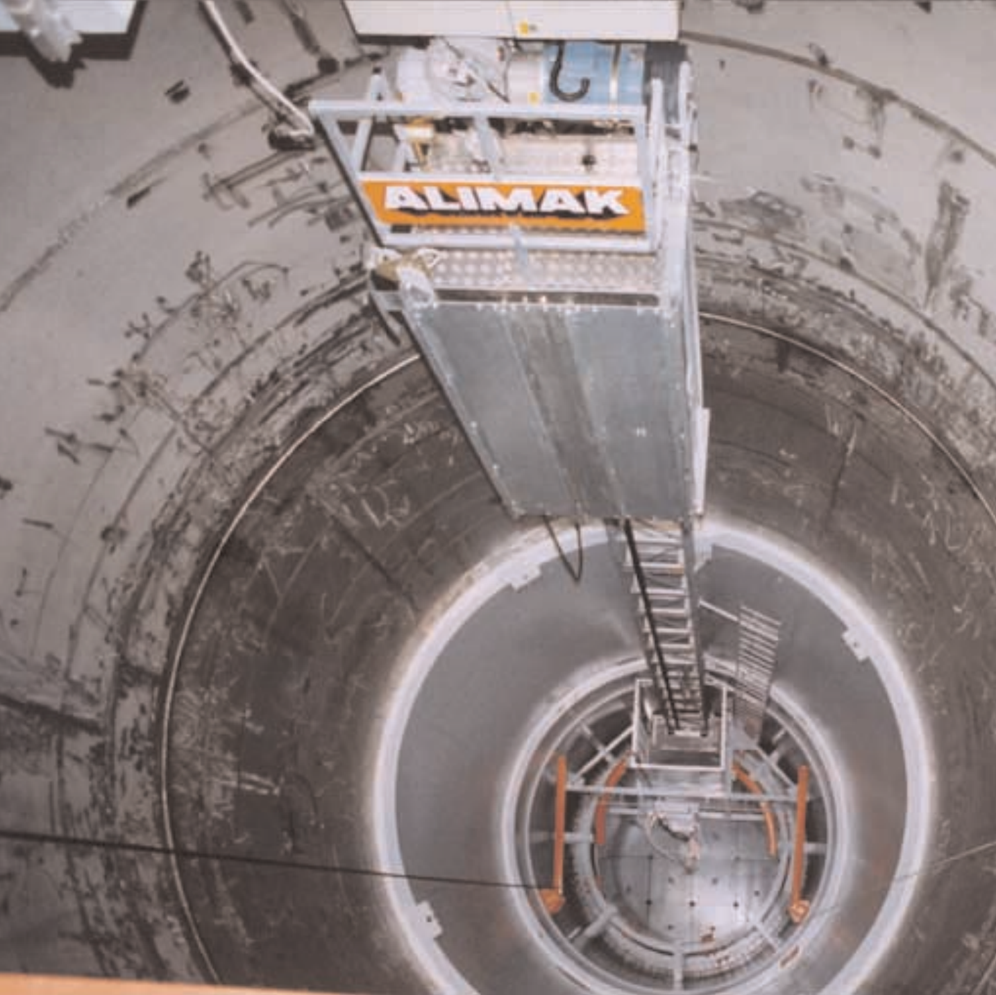
Photo: OKG AB, Project Fenix
