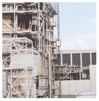
Alimak lift installation. This specific power station has 1 x 600 MW and 3 x 1000 MW boilers, and each boiler is served with an Alimak 10/19 lift, providing access to eight landing levels. The Alimak 10/19 lift fully complies with the Japanese Lift Regulations, providing a lifting capacity of 910 kg or 14 people.
