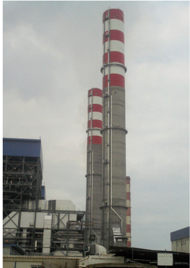
Two Alimak rack and pinion elevators gives easy access at the two chimneys for inspection and service.
