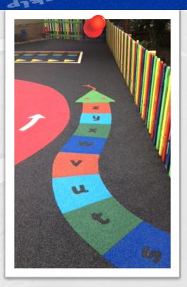
WET POUR RUBBER SURFACING is a bonded rubber surface designed for children's playgrounds and safety areas. Two grades of rubber crumb can be used, Styrene Butadiene Rubber (SBR) and Ethylene Propylene Di Monomer (EPDM). SBR is normally used as the base layer. SBR topping can release carbon so we do not recommend using SPR as a top layer. EPDM is the recommended topping layer and is available in black or other colours such as red, blue, green, yellow etc.'
