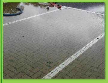
A corner area on a slight dip, caught water draining down the slope, yet that too drained within ten minutes of being flooded.
