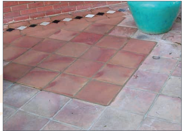
▲ These natural stone tiles were deep-cleaned, enhanced and sealed to restore natural hues also providing protection and ease of onwards maintenance.
