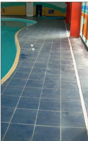
▲ A deep clean on a pool surround removing a calcium build up.
