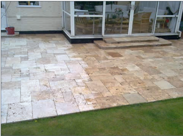
▲ These natural stone tiles were deep-cleaned, enhanced and sealed to restore natural hues also providing protection and ease of onwards maintenance.
