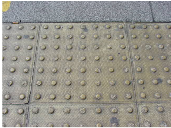
b) Pre-cast concrete blister tactile
