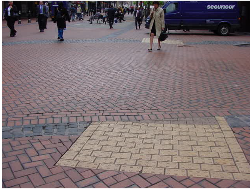
Figure 4.12 Uncontrolled crossing at the junction of New Street and Bennetts Hill, good colour contrast
