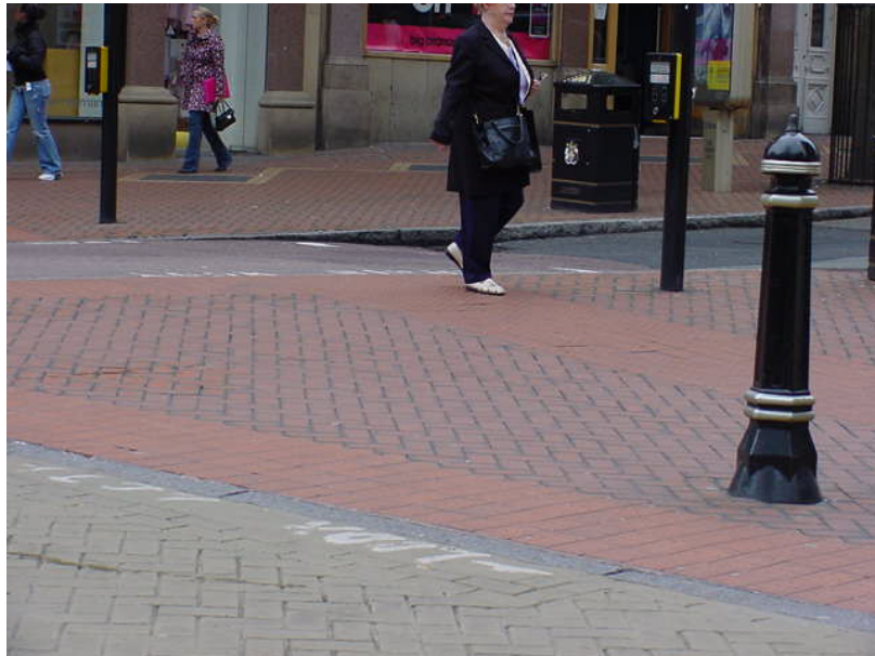
Figure 4.11 Controlled crossing on Corporation Street. Clearly showing lack of contrast between the tactiles and surrounding paving, note the lack of the contrast strip recommended in the guidance document.
