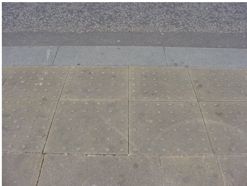
Figure 4.2 Peace Gardens uncontrolled pedestrian crossing. Tactiles used to indicate dropped curb. Tactiles made of the same stone as the surrounding paving so have no colour contrast.
