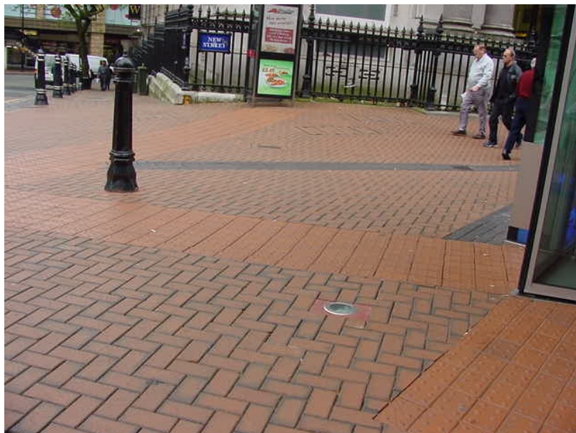
Figure 4.13 Junction of Corporation and Bull Street. Red block paving blister tactiles have been laid leading to a number of amenities.
