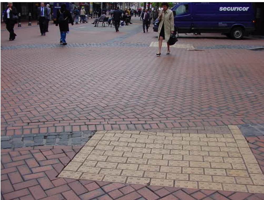
Figure 2.4 Photograph showing the correct use of blister tactiles at an uncontrolled pedestrian crossing.
