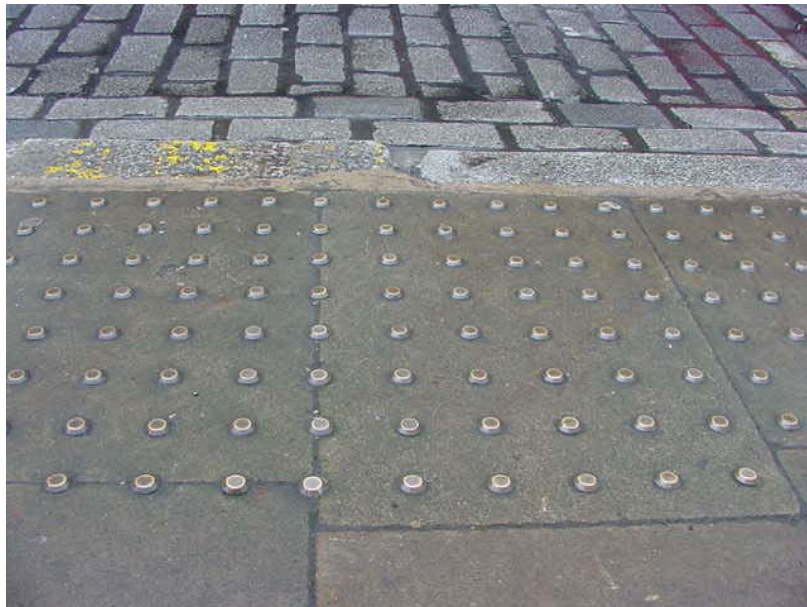
Figure 4.9 Detail of Upper Bridge Street uncontrolled crossing, showing brass studs set into existing stone paving.
