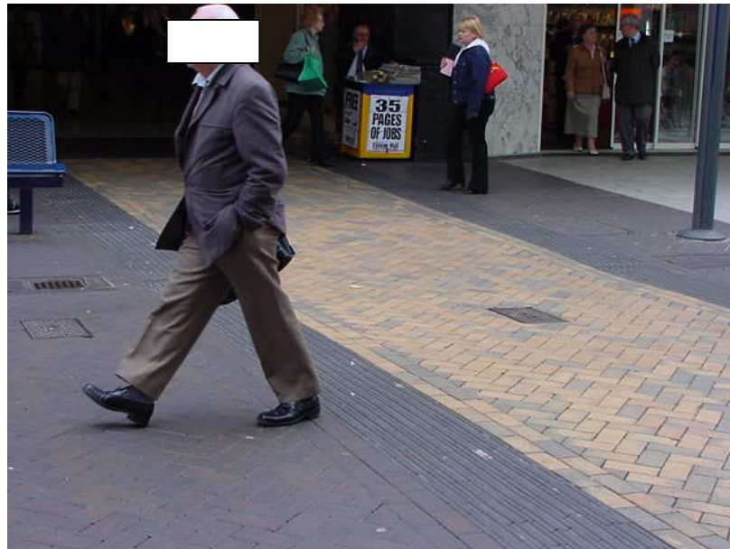
Figure 4.14 High Street corduroy tactile used to demark walkway into shopping centre crossing the pedestrianised area.
