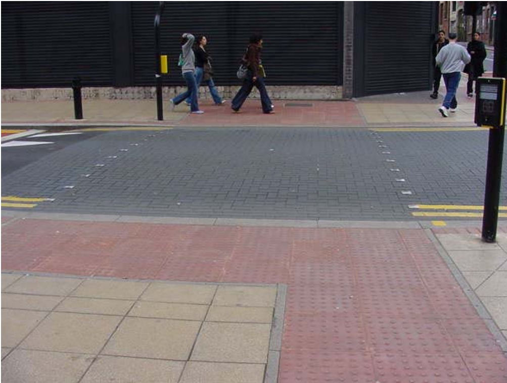
Figure 2.3 Photograph showing correct use of blister tactile paving at a controlled pedestrian crossing.
