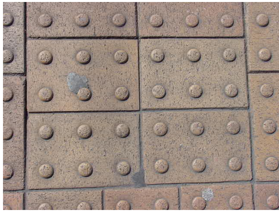
a) Block paviour blister tactile
