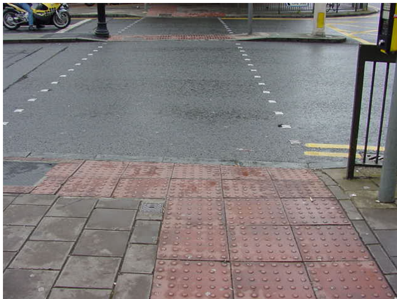
Figure 4.6 Junction of Grosvenor Street and Bridge Street. Tactiles installed to indicate controlled crossing. Correct use of tactile paving, good colour contrast with surrounding paving.
