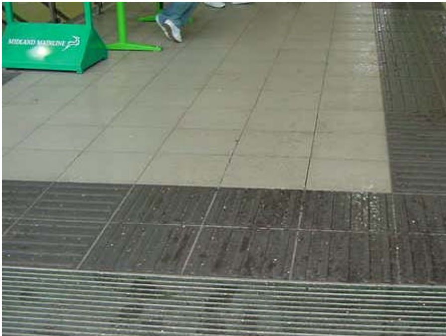
Figure 2.13 Example of correctly installed guidance path tactile, showing how easy it is to achieve good colour contrast with the surrounding flooring. In this example the tactile paving has been installed internally in a train station foyer.
