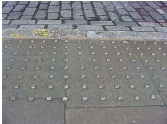
d) In-set brass stud blister tactile
