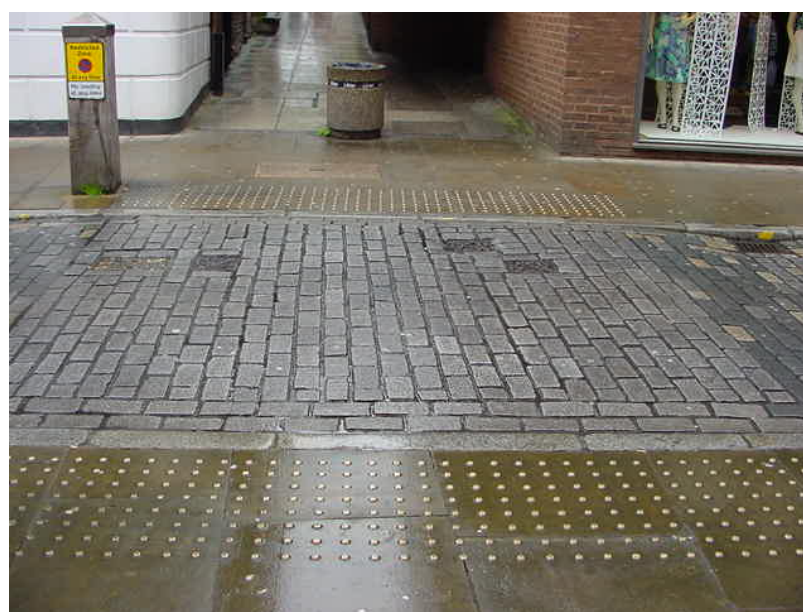
Figure 4.8 Uncontrolled crossing on Watergate Street. Brass studs have been installed into existing pavement. Right blister pattern, but no colour contrast with surrounding pavement.
