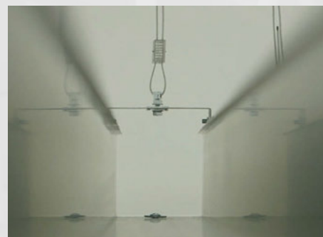
Image displaying adaptor and wire suspension in-situ, offering a mechanical fix to the services which are secure and level.
