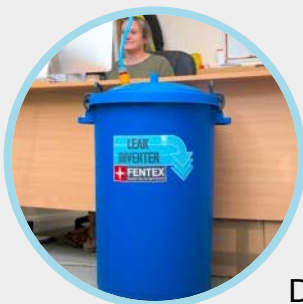
Fitted Drainage Point
