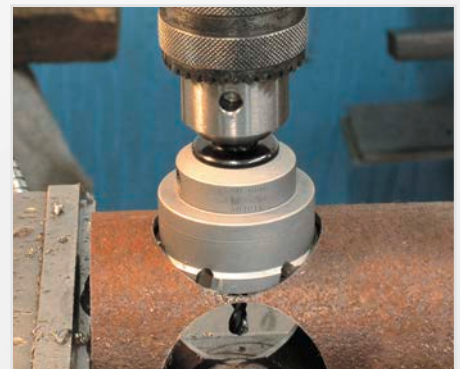
Drilling in pipes
