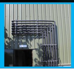
Chem Resist Pipework Systems Division are specialists in working with heat fused thermoplastics for handling corrosive solutions. Key advantages of the division are:-
