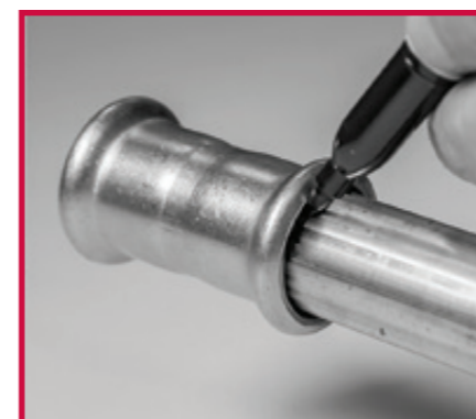
4. Rotate the tube and fully locate tube into the fitting and mark as shown for reference.
