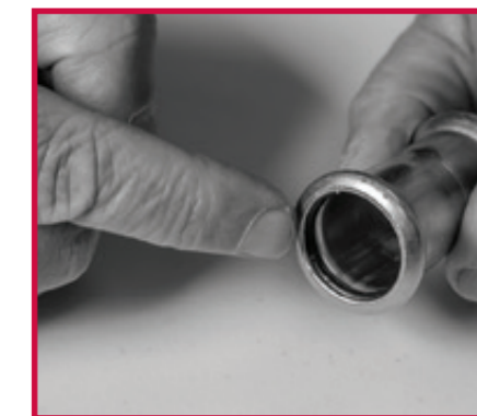
3. Ensure that the fitting O-ring is seated correctly. Do not use oil or grease.
