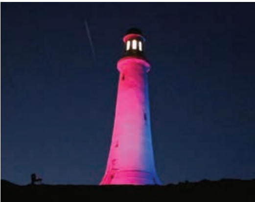
Sir John Barrow Monument, Ulverston, UK RGBW lighting installation with Wi-Fi
