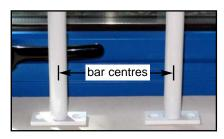
Now, using a tape measure, measure from the centre of your window out to the right ...at every 100mm point you'll need a bar (if it's a Child Safety Application), or at every 150mm for a security application. (Remember: the distance between the edge of the window and the centre of the bar closest to it should'nt be any greater than your chosen bar centres).
