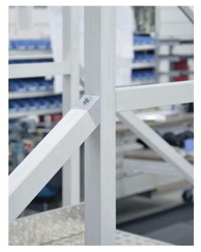
In a production plant for pharmaceutical products, a mobile bridge construction over a conveying path is required as part of the fire protection concept. The bridge must be made from non-flammable, cleanroom-compliant materials and must be non-slip. In addition, the bridge must be able to withstand a load of at least 240 kg and must not affect the transportation of products beneath it.
