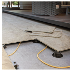
ON RAISED PEDESTALS SYSTEM
