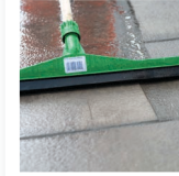
JOINTING MORTAR APPLICATION
