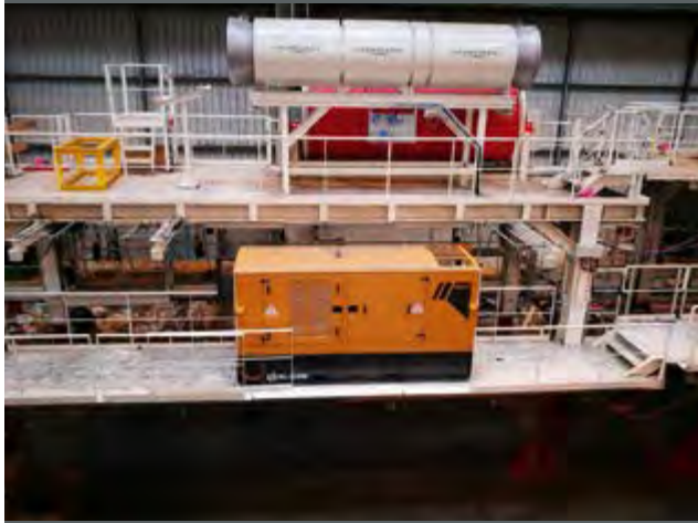
FRANCE - UNDERGROUND WORK 4 X GENSET 225/205 kVA
