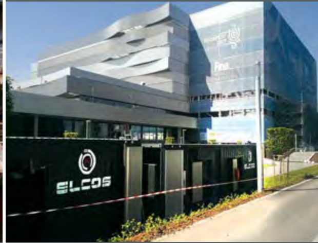
FINA HUNGARY 10 x NO BREAK Power Unit 40 kVA + 8 x NO BREAK Power Unit 20 kVA
