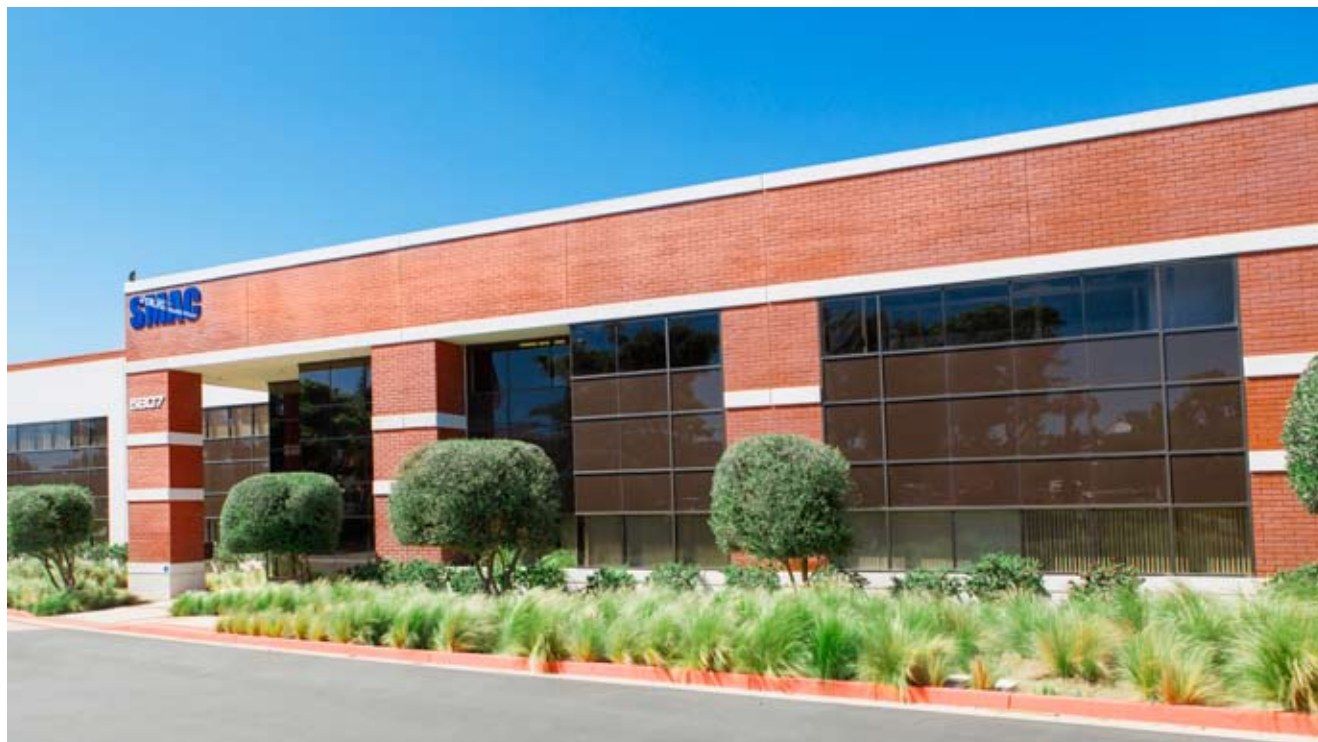
SMAC Corporate Headquarters and Factory
