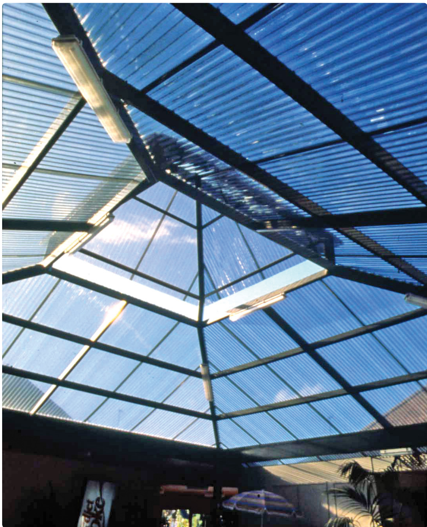
Project: Covered Patio - Denmark | Type: PALRUF® Clear 0.8mm
