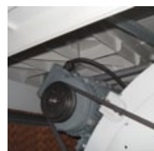
FAN WITH ANTI-CORROSION TREATMENT USING SPECIAL PRIMER AND RAL 7035 GRAY COLOUR.
