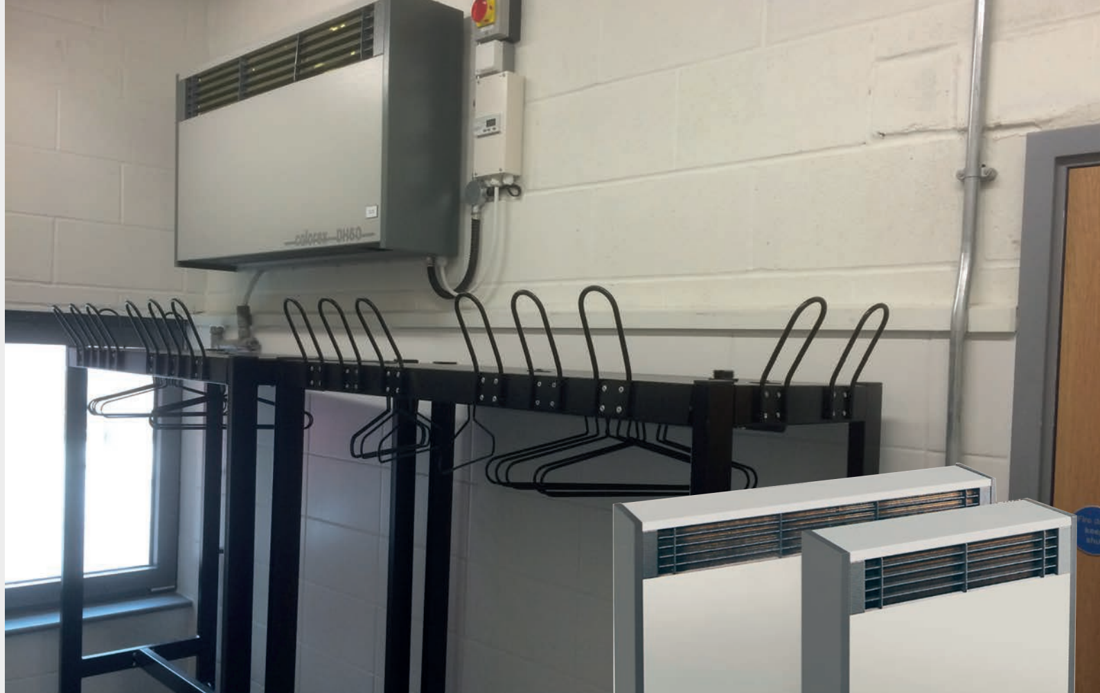
A Calorex DH60 installed in the drying room of Orpington fire station
