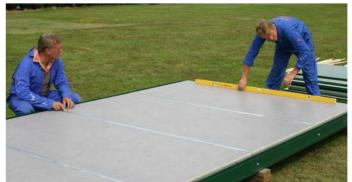
f. Site the chassis where you want to assemble the Cabin, check that the floor is level with a spirit-level, this is crucial for the smooth assembly of the unit.
