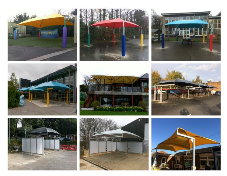
Fixed umbrella structures are an ideal alternative when there is little available area to install structural support posts. Umbrellas can be joined to cover almost any area & the gaps created between the structures are then closed with a flexible gutter joint to match the fabric roof. The steelwork support frame, the umbrella fabric & the bumper pads can be supplied in multiple colours to create a superb eye-catching finished product
