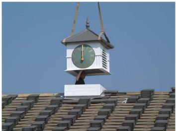
Cupola being lowered in to position. The use of a crane is recommended on cupolas over 900mm wide.
