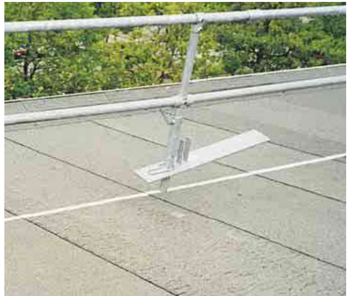
Full edge protection is maintained during refurbishment and repair work.
