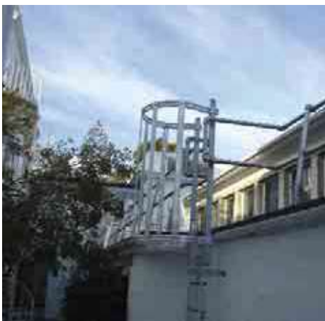
Cat ladder installation connection featuring guardrail return connection
