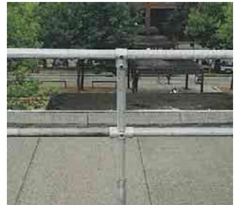
In Line 'T' Connection This method uses cast 'T' pieces to connect the handrail tubes in the same plane as the vertical post.
