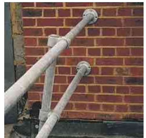
Wall Plate Fixing
