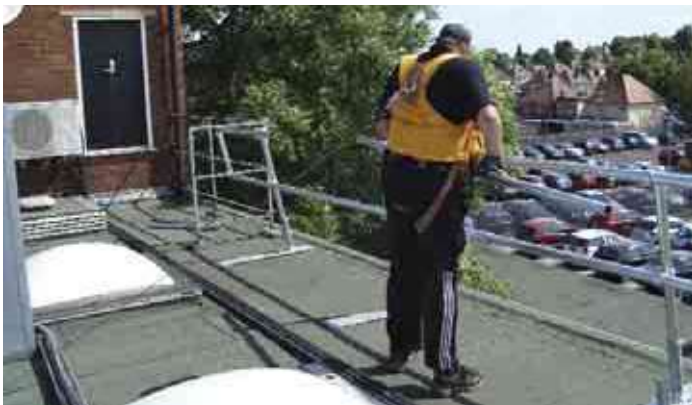
Final stage of guardrail installation.
