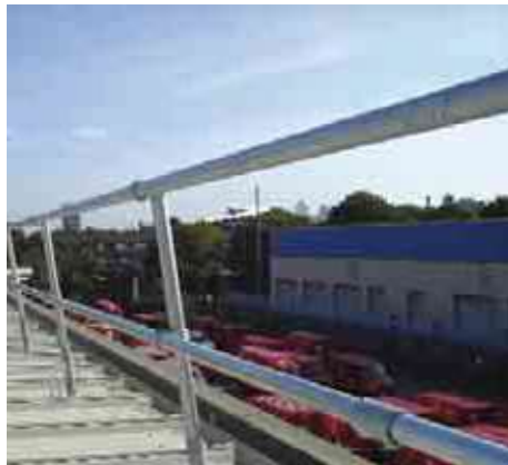
90° Crossover Clamp Connection This method uses cast clamps for fixing handrail tubes to vertical posts. The system can be used safely on metal profiled sheeting.
