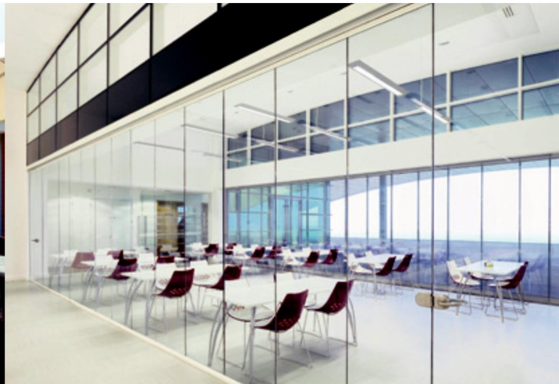
View of Manchester United's training ground staff restaurant with single-glazed curtains and restaurant extension with double-glazed curtains
