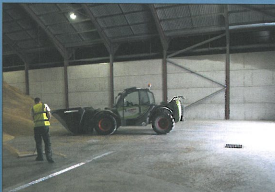
Prestressed concrete wall panels are robust, durable and easy to clean.
