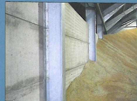
Division walls can be constructed using double loading horizontal panels fitted between column webs (above) or using freestanding vertical cantilever panels cast into the floor slab (below).
