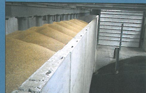
Division walls can be constructed using double loading horizontal panels fitted between column webs (above) or using freestanding vertical cantilever panels cast into the floor slab (below).
