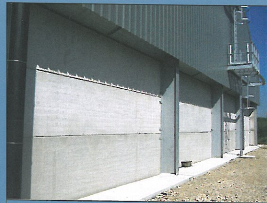
Panels use a simple clip system to fix to the building.
