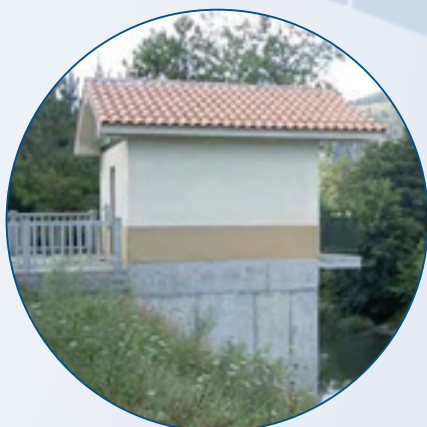
Measurement station, built to specification and fully equipped
