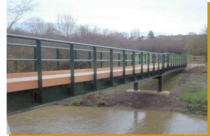
Painted steel beams and metal fabricated parapets
