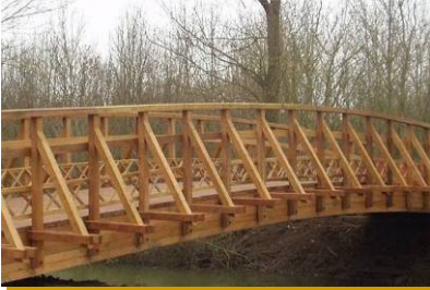
Steel beams clad with a hardwood fascia
