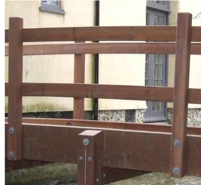
Type B parapet
