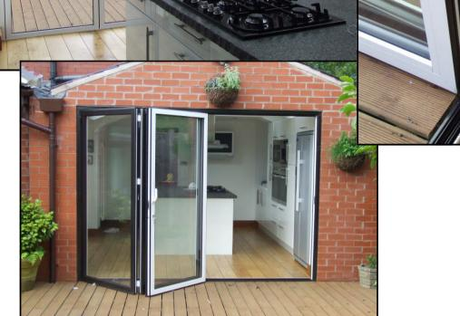
Weathered track built in to the floor to give a low threshold between the inner and outer levels while maintaining an effective weather barrier
