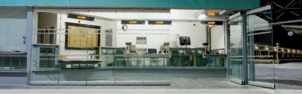
The fully glazed MSW glass-to-glass system installed at the Travel Centre in Chester Railway Station creates a transparent frontage that combines ease of access, security and full visibility. This combination makes the MSW suitable for use in high traffic, public locations. At seven metres long, the wall can be fully or partially opened as required. The glass modules move easily and quietly on ball bearing suspensions running in an aluminum track and stack neatly at one end.
