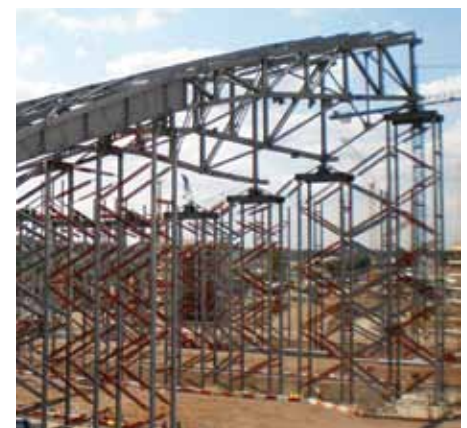
Engineering solutions for the impressive 2010 Olympics Aquatics centre roof
